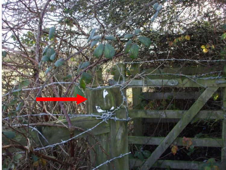
The Rixon Gate end of the claimed route, former kissing gate access, now wired shut, with remnants of waymarking disc. Photograph taken by Janice Green, Rights of Way Officer, January 2018.
